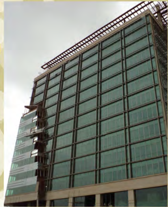
Installed Systems - Indoor Units
